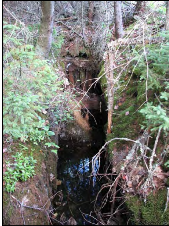
PLATE 20: Wooden bracing within an exploratory gold mine shaft at Area 11. Facing southeast. September 15, 2014.
