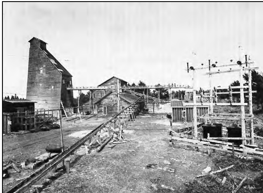
PLATE 11: Mining facilities at Montague Gold District in the early twentieth century (Bates 1987: 13).
