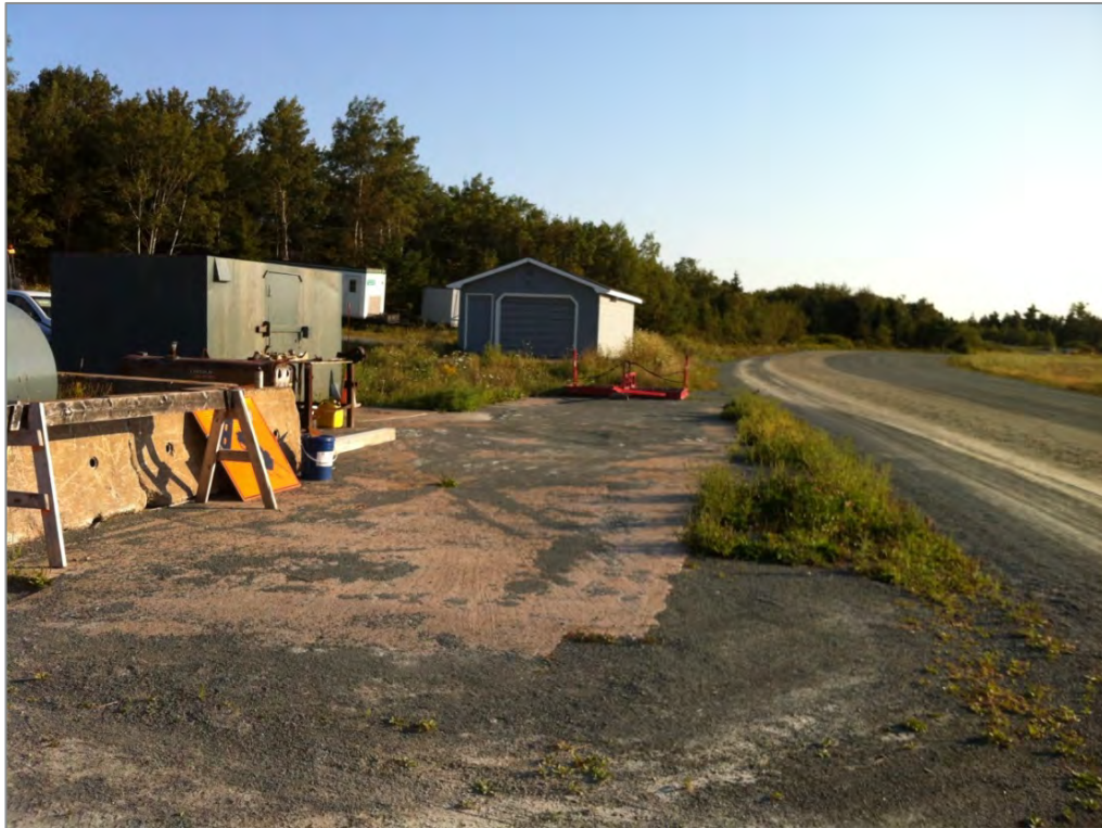
Image 3.5-2: Site of building fire several years ago, next to an AST, August 26, 2014
