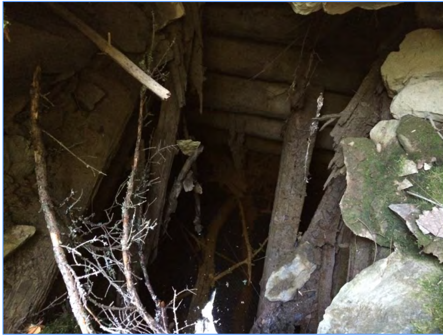
Photo 10: Abandoned mine shaft, adjacent to Study Area
